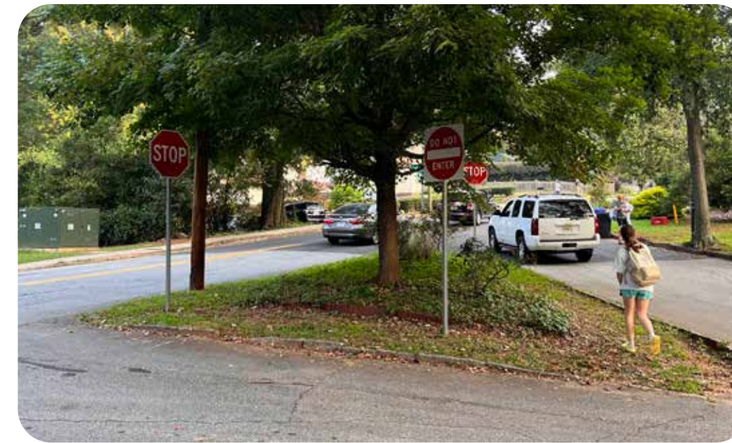
No clear pedestrian crossing route and numerous conflicts due to the slip lane
