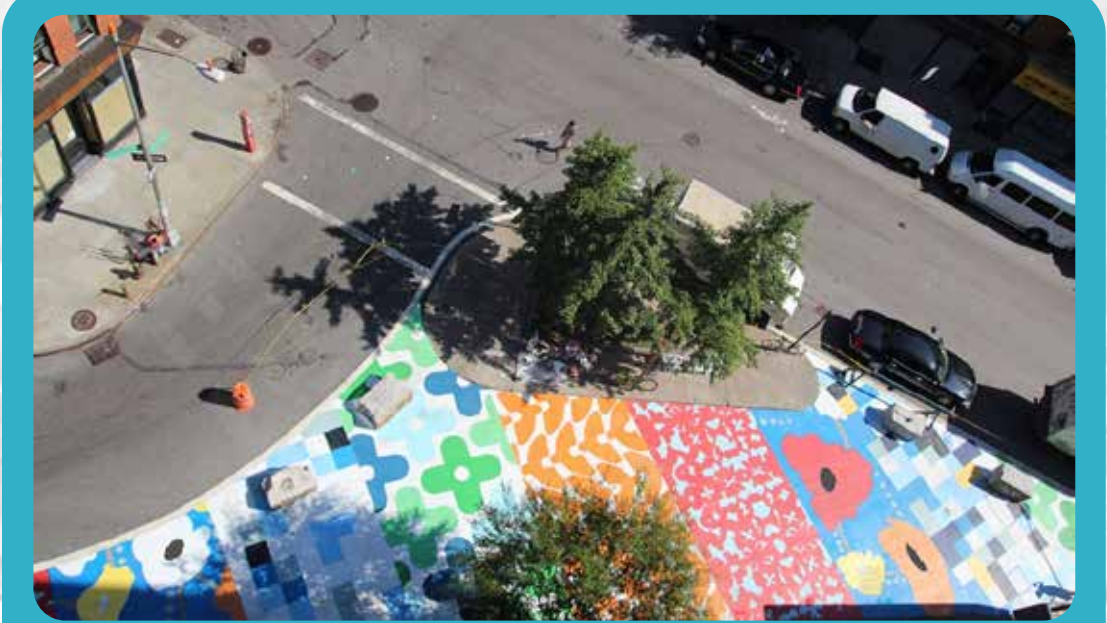
Slip lane closure with neighborhood mural opportunity protected by flexposts and wheel stops; better organizes the intersection to direct pedestrian crossings, increase pedestrian visibility, and reduce vehicular speeds
