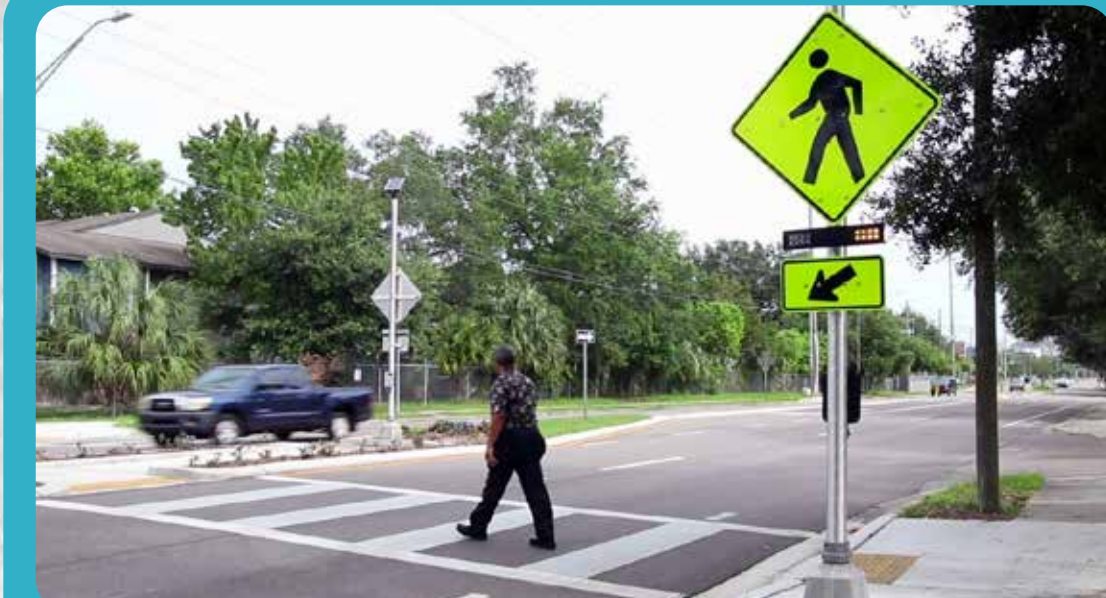
New pedestrian crossing with rectangular rapid flashing beacons (RRFBs) to provide a predictable, safe crossing for pedestrians along the existing sidewalk on S McDonough St (new sidewalks are outside the scope of this project), increase crossing visibility to drivers, and to reduce vehicular speeds; crosswalk is also a potential asphalt art/mural opportunity
