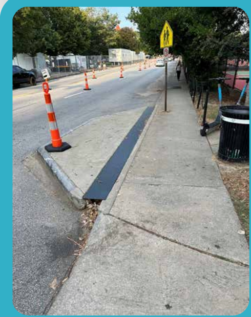
Curb extensions to protect pedestrian crosswalks, increase visibility, improve driver attentiveness, and maintain stormwater drainage patterns
