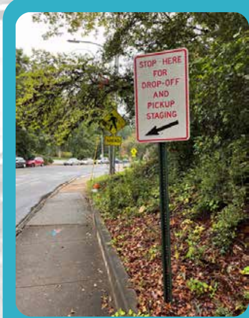
Adjust curb location and provide new signage and stop bar to increase pedestrian separation from the street and guide the drop-off queue to keep the intersection clear for large, right-turning vehicles
