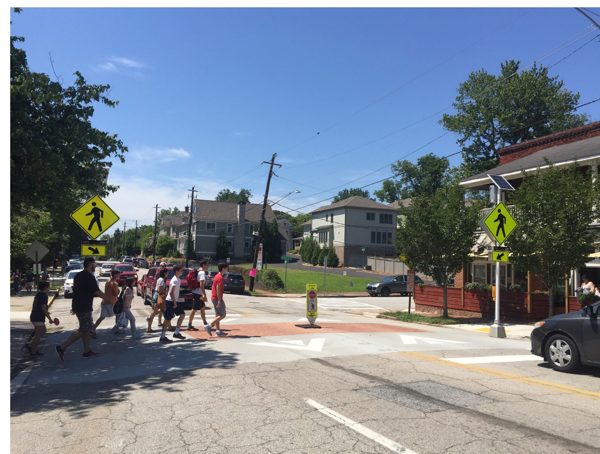
PEDESTRIAN CROSSING WITH RAISED CROSSWALK
